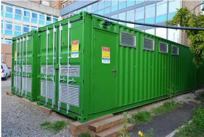
and rapid solution which the hospital needed. The containers are currently positioned adjacent to the Maternity building but could be moved at any time to an alternative location to suit future site development plans. The containers have been thermally and acoustically treated and fitted with purpose designed ventilation. Fire detection is installed within each container and linked to the central hospital system. Self-contained emergency lighting units are installed in each container.
