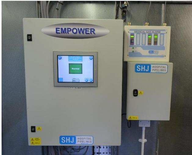
These innovative controllers, developed by SHJ Hospital Pipeline Systems, interface with all aspects of the medical gas plants ensuring optimum operational performance and maintaining a log of plant operating data. Plant status can be remotely monitored allowing early initiation of any remedial action needed.
