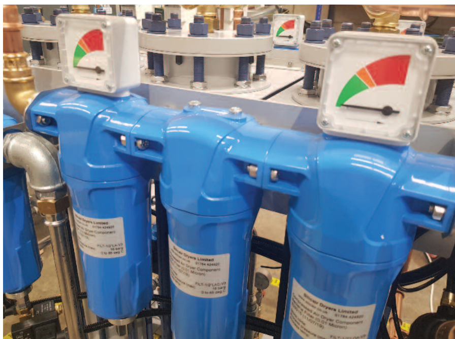
The Silicair medical air driers, which use 'a special desiccant mix, which includes a substance used to convert harmful carbon dioxide from car exhaust fumes to CO 2 '.
