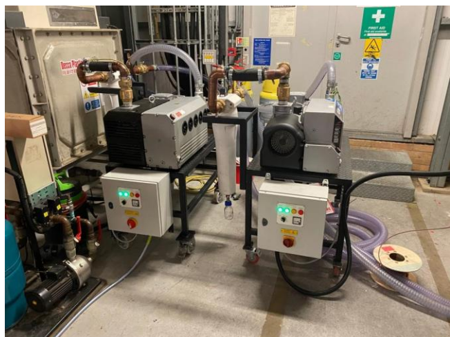
SHJ temporary plant, which keeps hospitals fully supplied with medical gases during installations.
